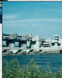
Lock and Dam
