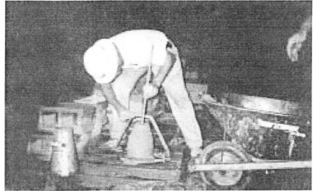
Fig. 2.1—Initial concrete slump before the addition of HRWRA.
