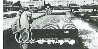
Hollow-core, pre-stressed concrete panels.
