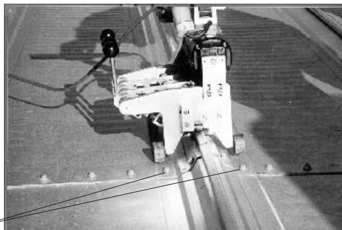
Photo 3B Electric Seaming at Endlap
